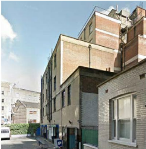
Street view of the south elevation
